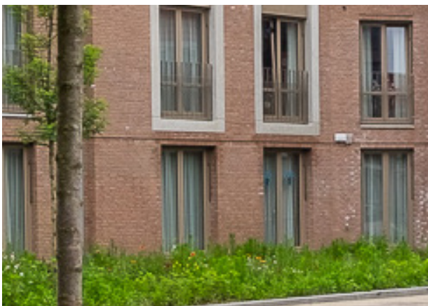
French balcony with French door to create private outdoor space F Ground level; French doors with small greenery as 'fence' G
