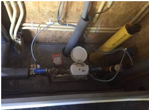
Figure 2.3 Smart meter attached to and installed in front of the normal water meter at a household
