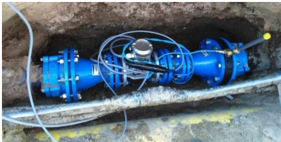
Figure 2.1 Example DMA inlet meter
