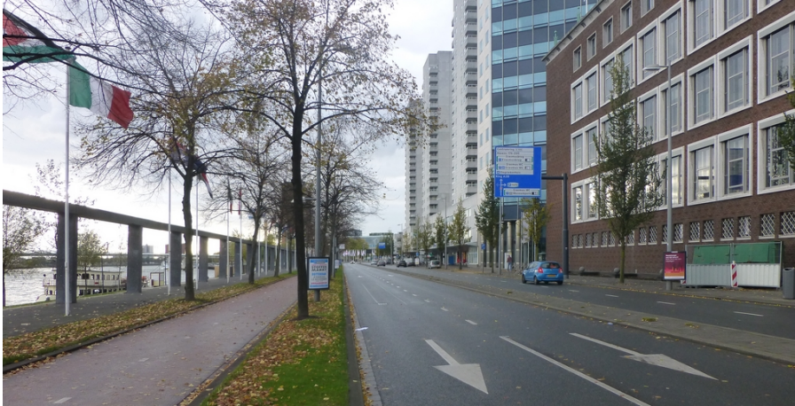
Figure 6.26: Rotterdam: the Boompjes seen in western direction, November 2016
