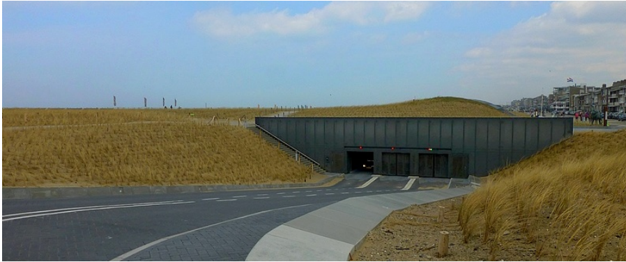
Figure 6.10: Katwijk: car entrance to the underground parking garage. The dike is embedded in the dunes (on left side of the picture, hidden under the sand), May 2015
