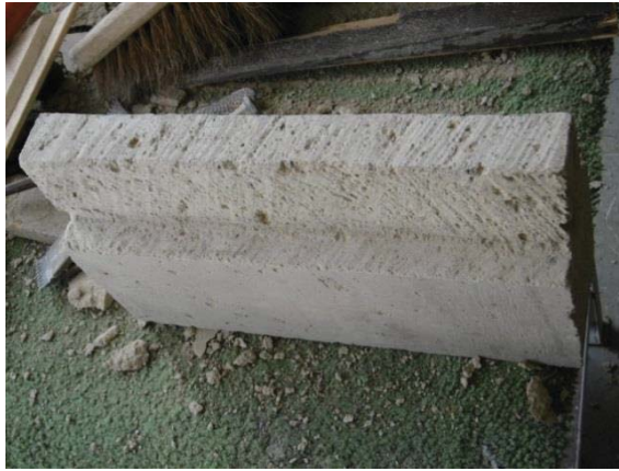
Fig. 5. Example of a tooled mullion.
