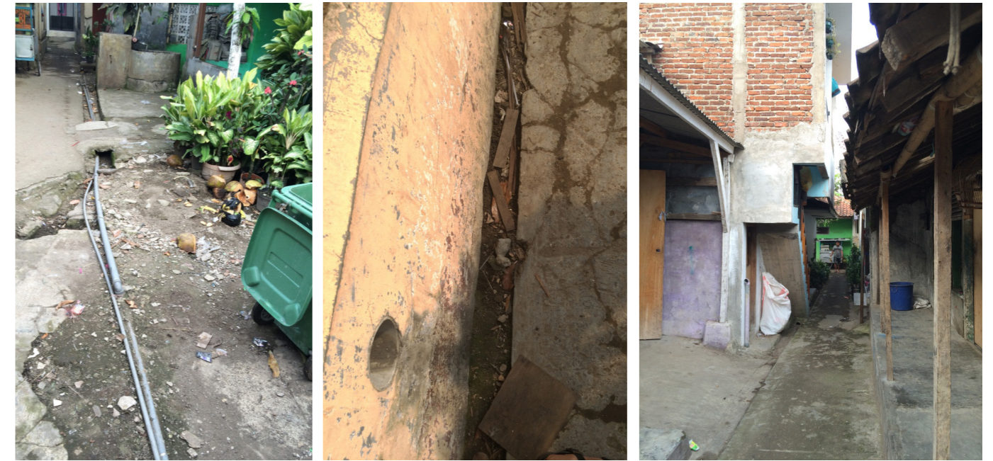
Figure 20. Concrete covered alleys with unorganized water pipes (Own illu.)
