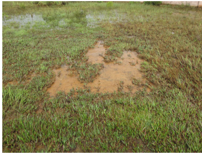
Figure 6.5: Damage at the YB3 dike toe after 60x4 + 80x6 + 100x4.
