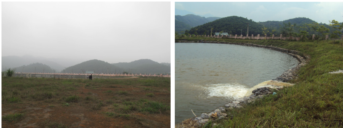
Figure 1.1: Site of constructing the super dike model and the water source.
