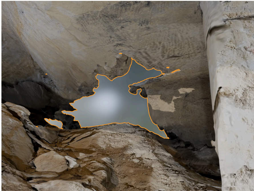
Figure 2.5: Some of the empty polygons in ZW3-pillar. The missing polygons are enclosed by the orange line. Own work.
