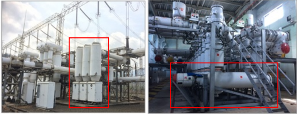
Figure 1.5 Two examples of 500 kV GIS of the JABA case study. Both GISs have a single phase per enclosure design. In the left figure, the outdoor GIS has a vertically designed CB, while in the right figure, the indoor 500 kV GIS has a horizontally designed CB. CB is shown by the enclosed red box.
