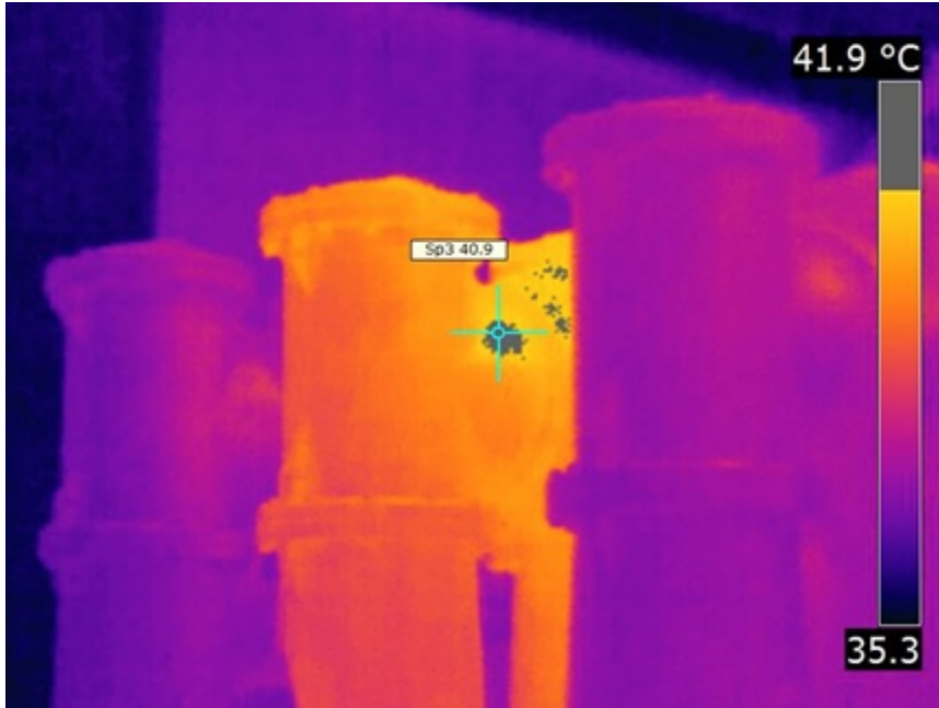
Figure 4.8 An example of a hotspot in one phase of sealing end compartment in a GIS in the case study. The thermal image camera captured the picture. The highest temperature point is indicated by the “plus” symbol in the picture. Further investigation reveals the degraded jointing of the primary conductor at that point.
