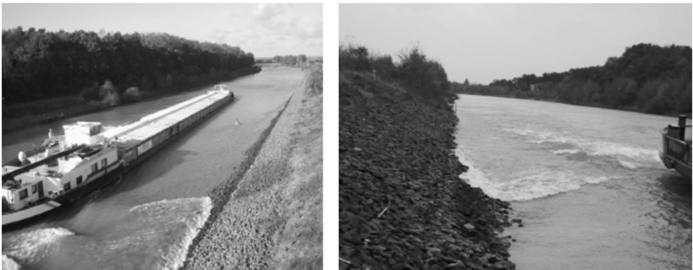
Figure 4.25: Stern wave breaking on a bank (images by Bundesanstalt fr Wasserbau (BAW) are licenced under CC BY-NC-SA 4.0).
