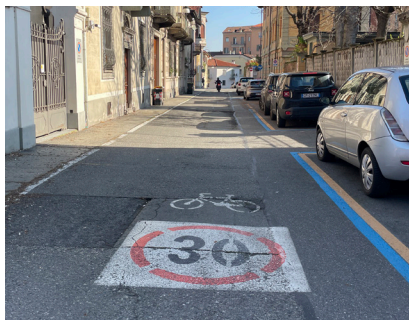
Figure 3. Shared-use route within traffic-calmed zone 30 area. Photograph by the author. Field observation, Turin, March 2026.
