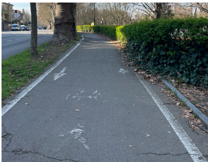
Figure 11. Poorly maintained path (faded markings, uneven surface). Photograph by the author. Field observation, Turin, March 2026.
