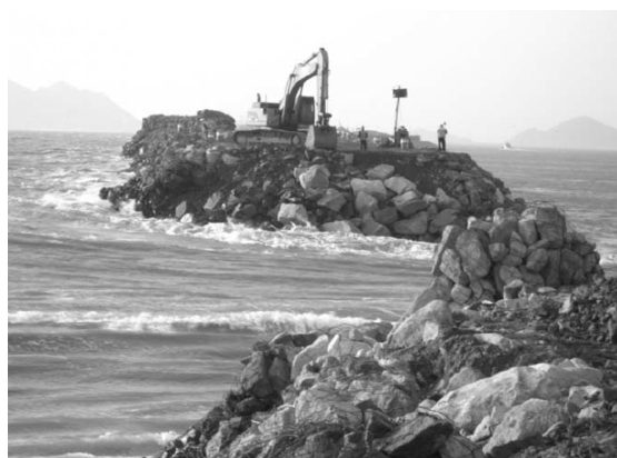
Figure 6: Construction of a rubble mound breakwater
