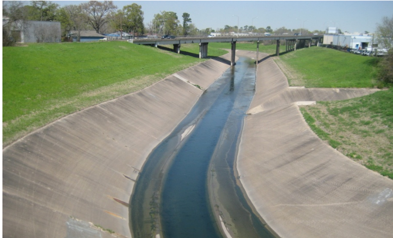
Figure 13: Flood channel Houston, Texas, US
