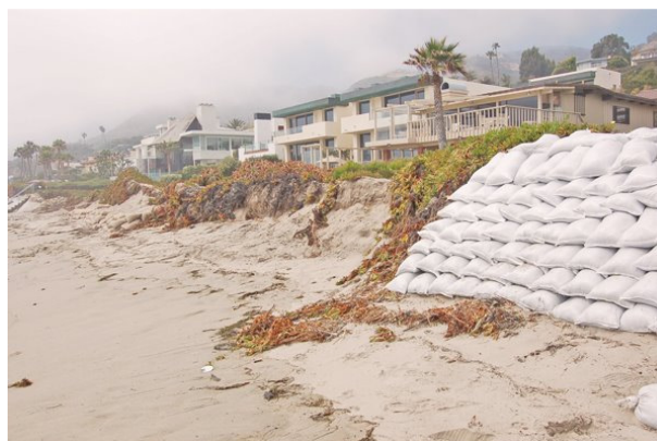
Figure 12: Sandbag protection
