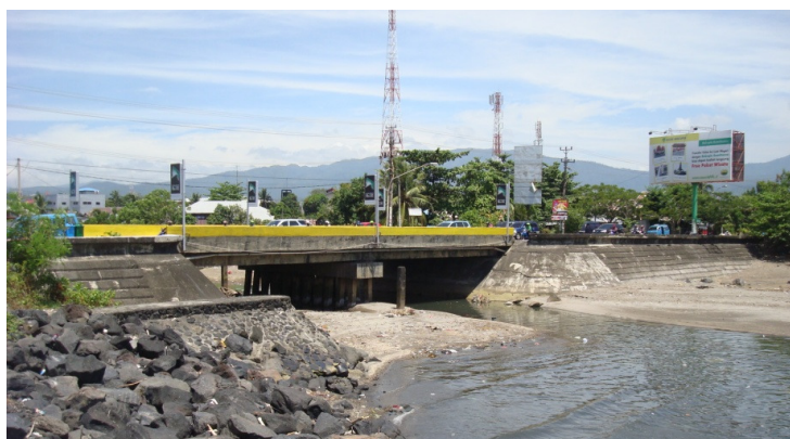
Figure 6: Photo of the Sungai Sario outlet
