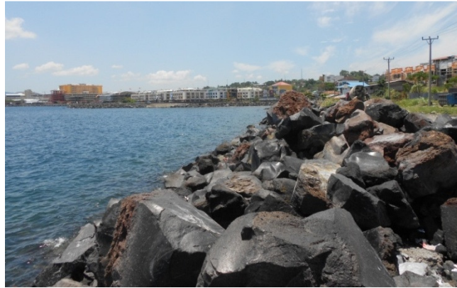
Figure 7: Rubble mound protection
