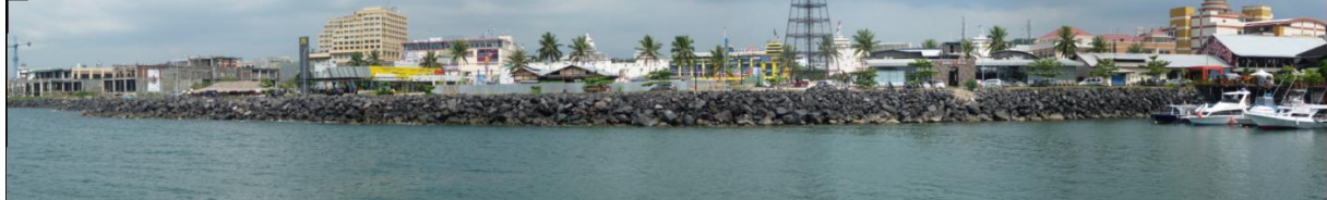
Figure 7: Coastal protection at the beach site
