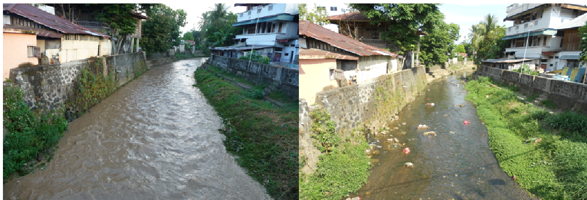
Figure 15; Upstream of bridge (L), downstream of bridge (R)
