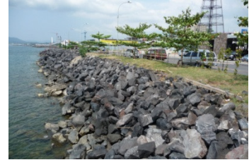
Figure 10: existing coastal protection
