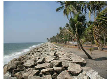
Figure 14: Rubble mound protection
