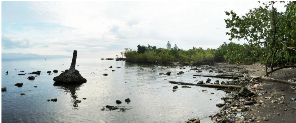
Figure 2: Erosion near Molas
