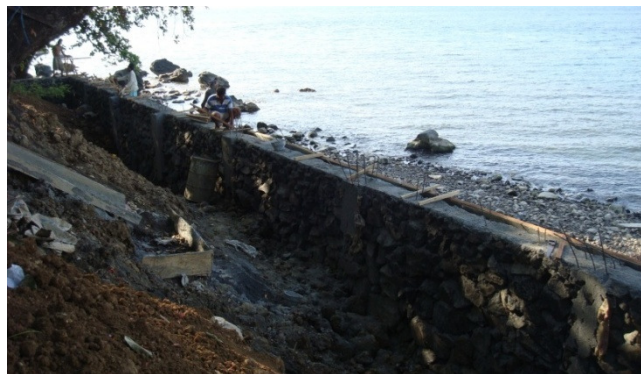
Figure 4: Protection under construction
