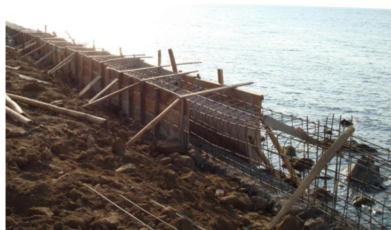
Figure 5: Wall under construction
