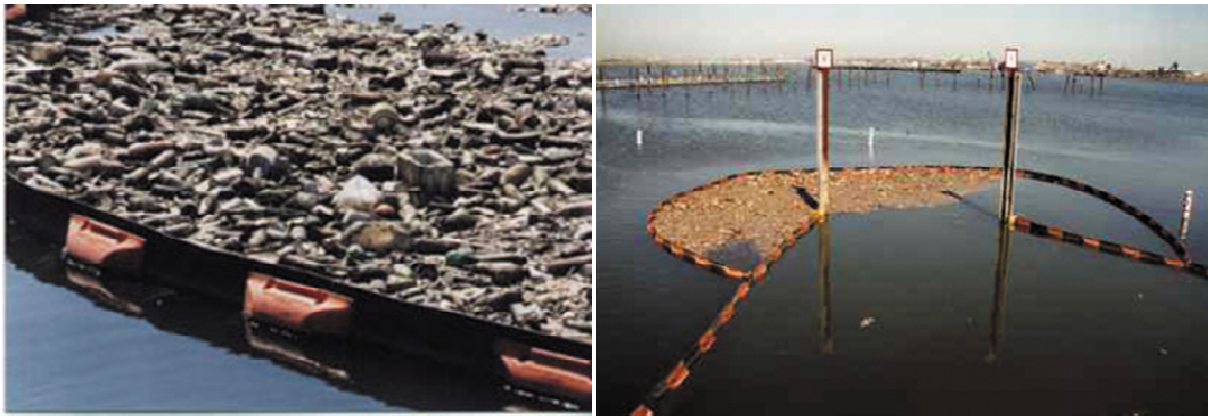
Figure 6: Garbage catch structure
