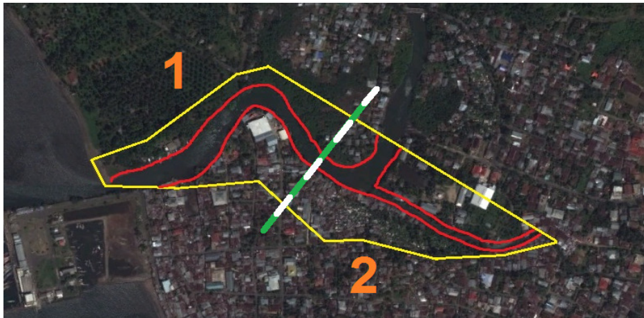
Figure 1: Tumumpa flood area
