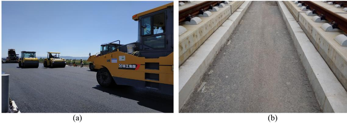
Fig. 2. The asphalt supporting layer (ASL) in test section: (a) Under construction, (b) In operation.
