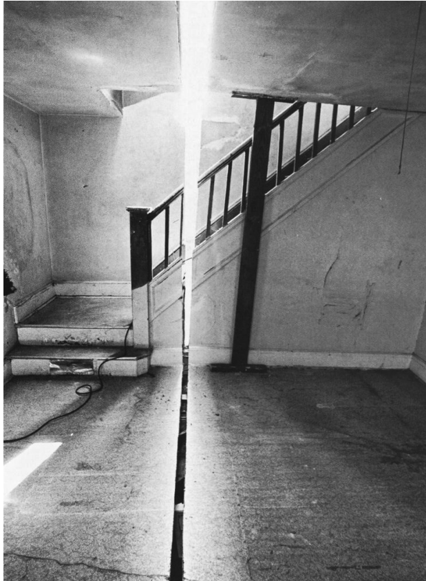
splitting intervention, gordon matta-clark, englewood, 1974
