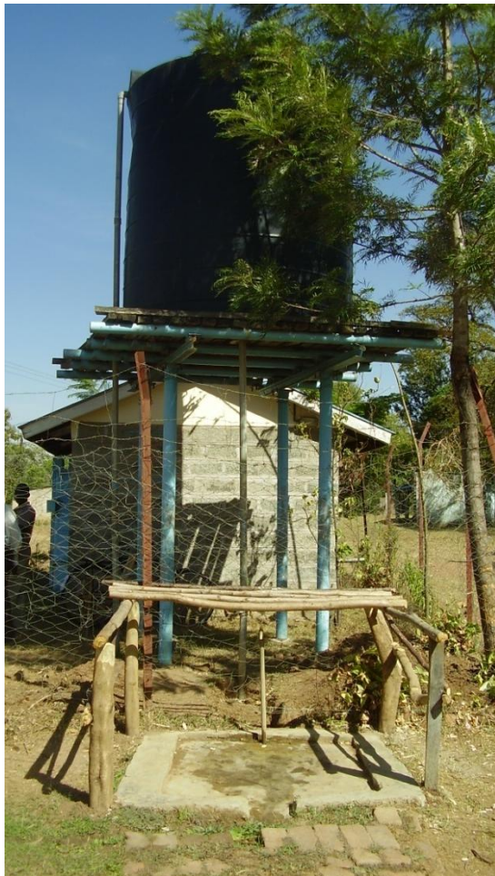
Figure 2.8 Water supply from motorized pump with elevated tank, generator house and tap (picture A. Adams)
