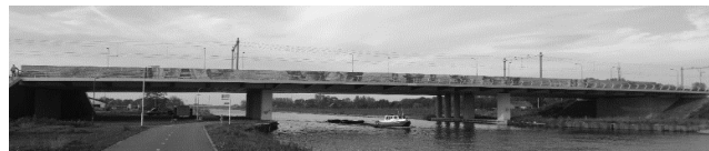
Figure 18. Monitored railway bridge in Rosmalen.
