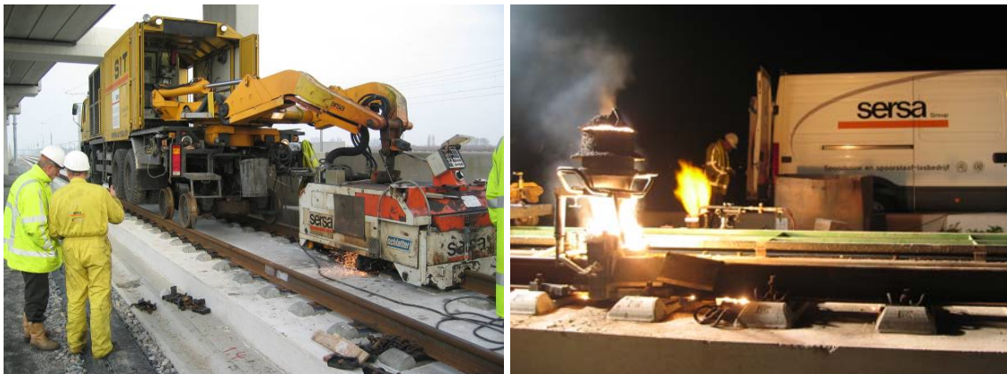
Fig. 4.2 Flash butt (left) and aluminothermic (right) rail welding on the Dutch HSL-South (courtesy: Wijnand Paans, BAM Rail)
