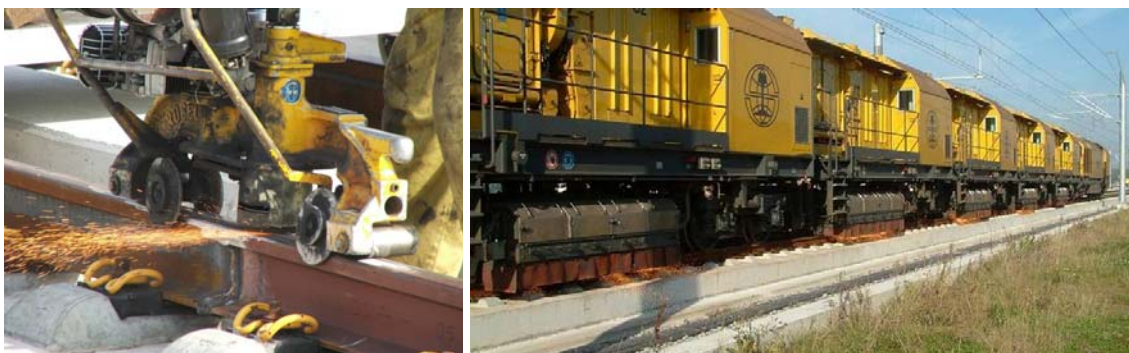
Fig. 4.3 Manual rail weld grinding (left) and grinding train (Speno) (right) on the Dutch HSL-South
