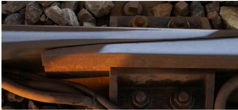
Fig. 1.13 Rail transition in an expansion joint
