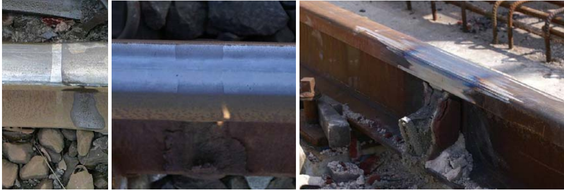
Fig. 4.4 Weld and parent material (left: flash butt weld; centre: thermite weld); the heat-affected zone after thermite welding and grinding (right)
