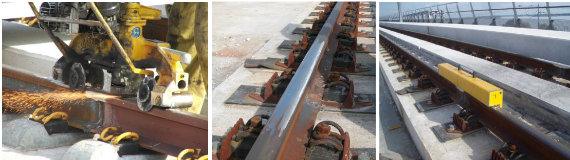
Fig. 4.61 Semi-mechanical grinding of the rail weld surface in longitudinal direction, ground rail and electronic geometry measurement
