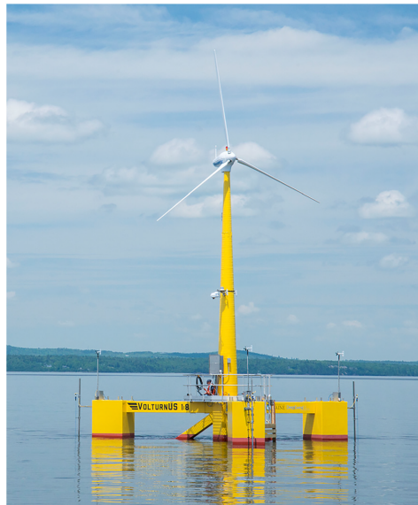
Figure 2.2: VoltornUS 1:8 scale prototype [7]
