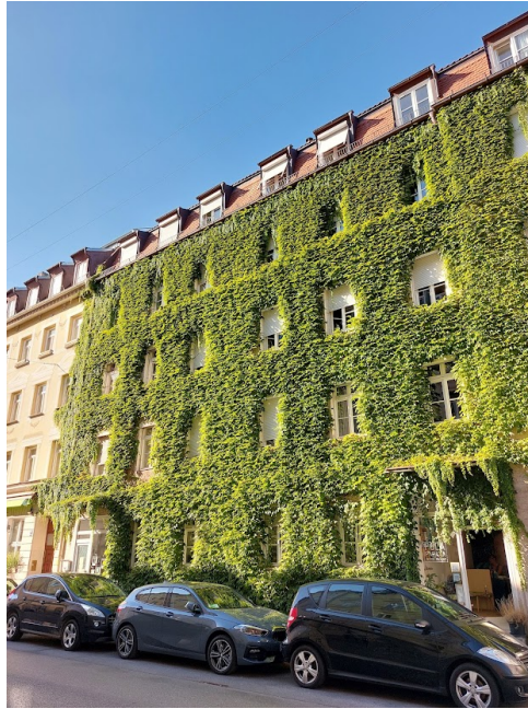
Figure 4.2: Direct green facade (DGF) in Munich (own work)
