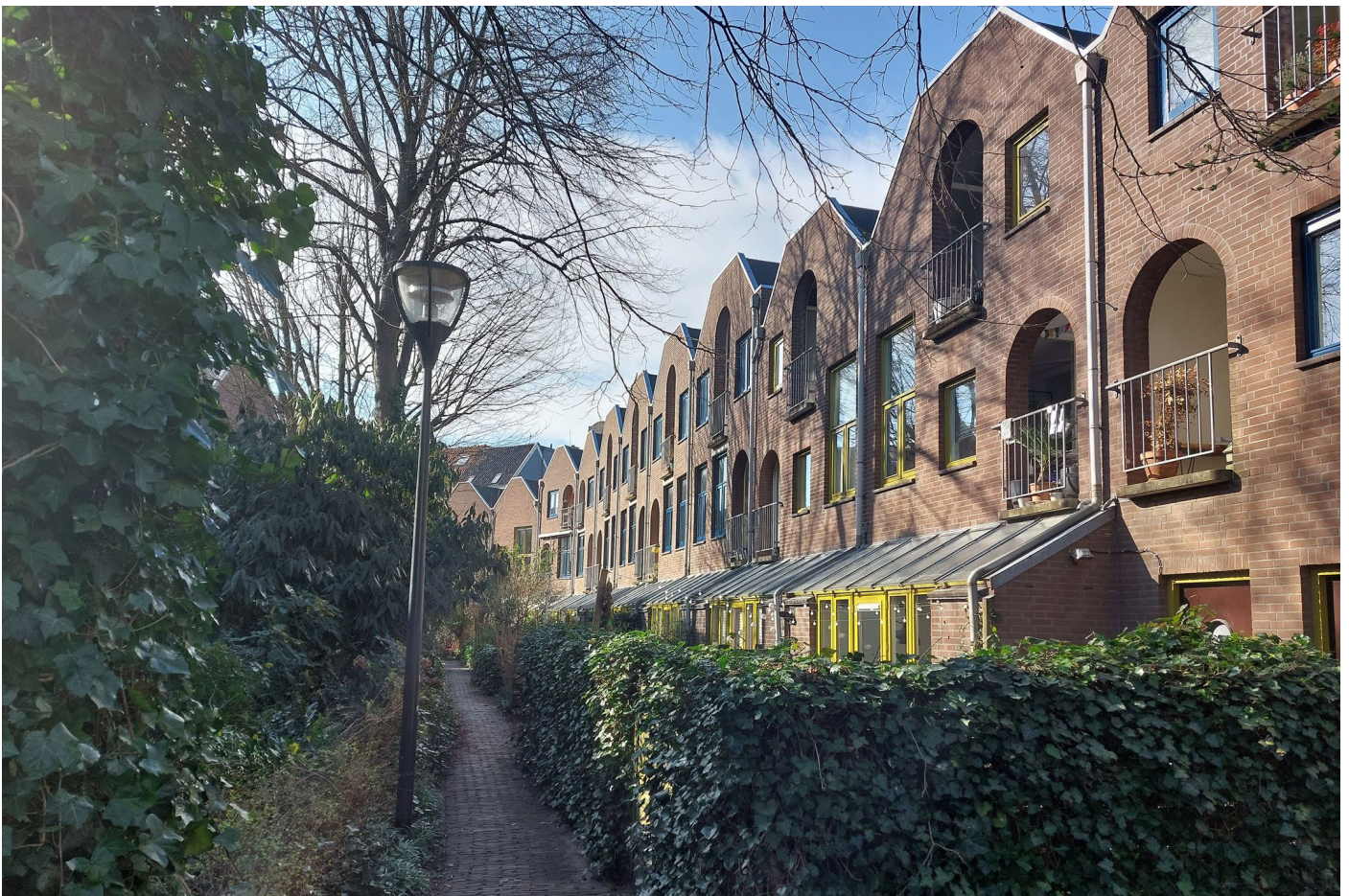
Fig. 40 Urban renewal project 'Onder de Bogen', Zwolle by Theo Bosch and Aldo van Eyck (Funda, 2022)
