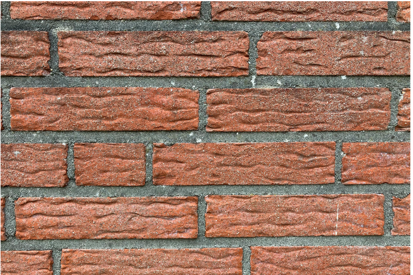
Fig. 55 Brickwork Goedewerf (photograph by author)
