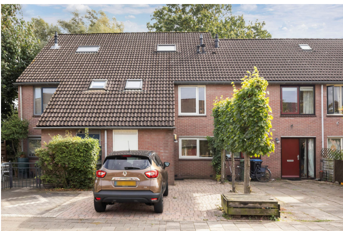
Fig. 31 Large amounts of roof area. Verenwei, Arnhem (Funda, 2022)
