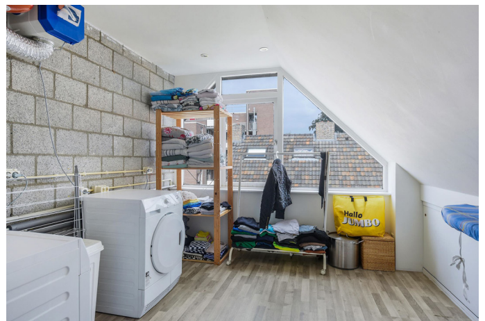
Fig. 30 High quantities of thermal mass: loadbearing structures made of concrete or brick. Dapperstraat, Tilburg (Funda, 2022)
