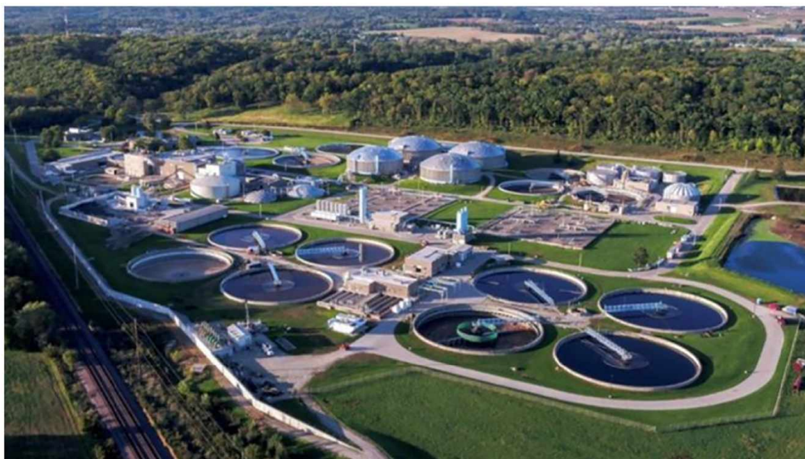
Figure 7 | Cedar Rapids Water Pollution Control Facility.
