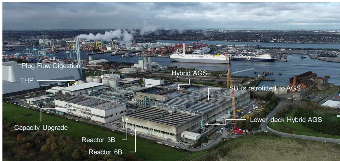
Figure 5 | Ringsend WWTP with retrofit to AGS nearing completion. Reactor 3A was already retrofitted into AGS in 2017 (in former SBR 3B) and used to validate performance of AGS and hybrid AGS in former SBR 6B (bottom). Source: Modified from Buyers-Basso (2024).
