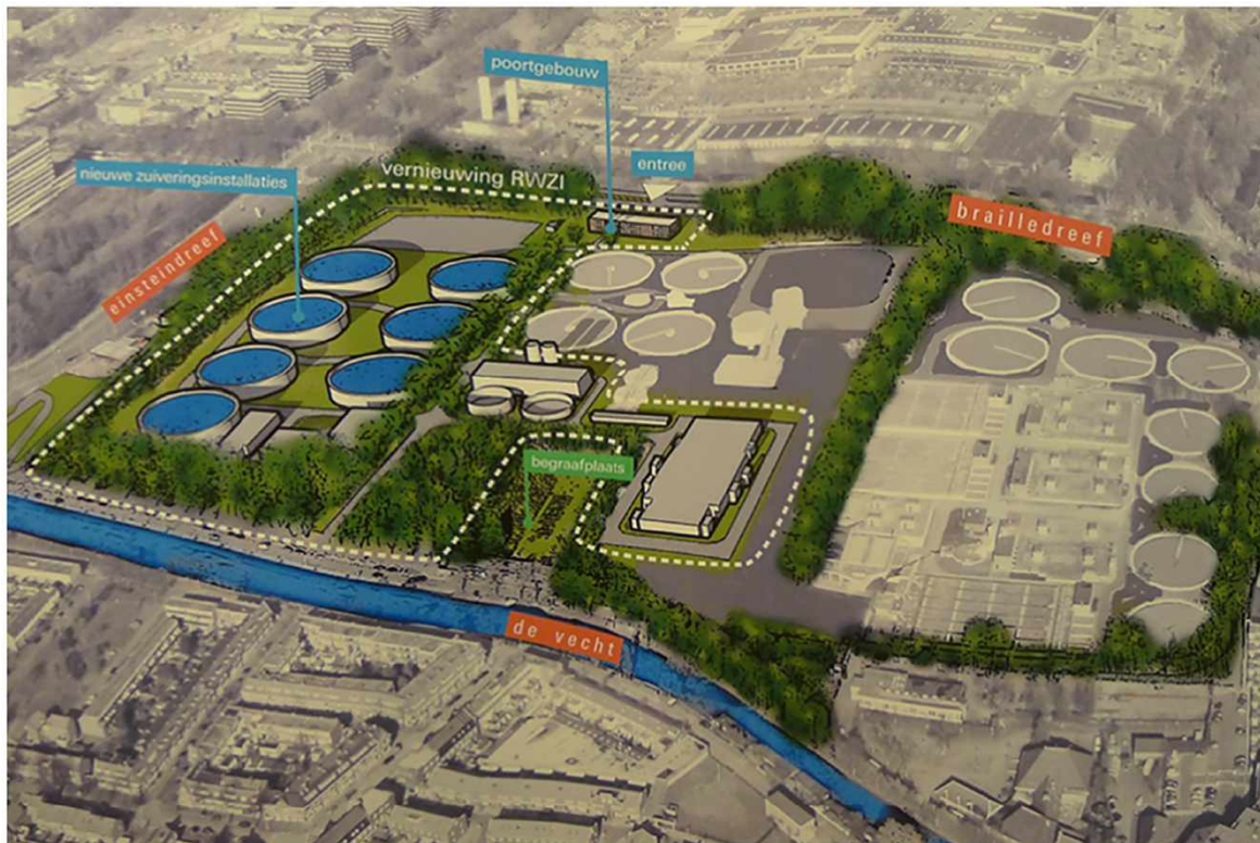
Figure 3 | New AGS-based WWTP of city of Utrecht (dotted area left) projected on decommissioned activated sludge infrastructure (Source: www.Nereda.net ).
