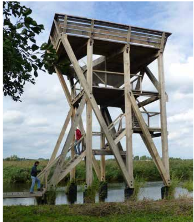
FIG. 1.2 Watchtower Kalverpolder, Zaandam. Daf-Architecten, 2013. The design is inspired by the construction technique of the windmills in the region.
