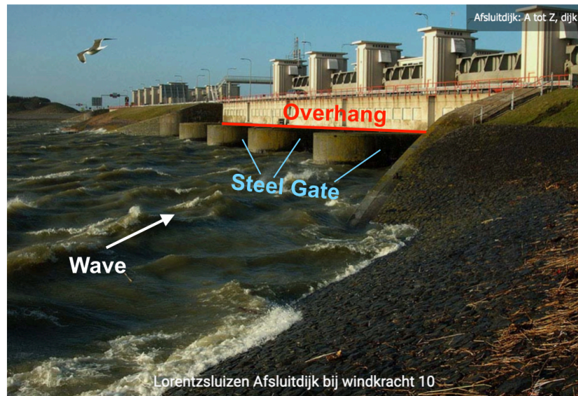
Figure 1.3: Stevin Outlet Sluis (Afsluitdijk), One typical vertical structure with overhanging (Kees Looijesteijn photography)
