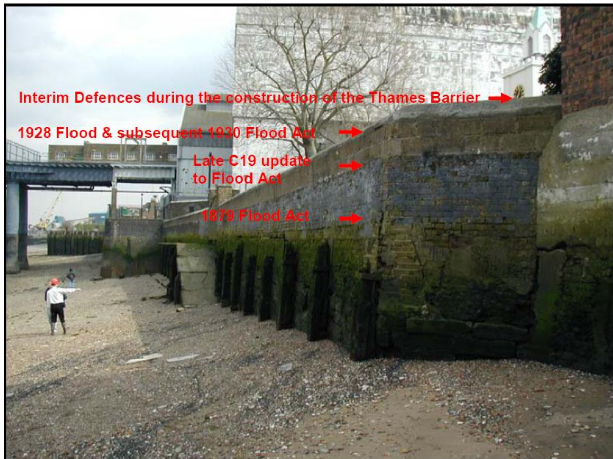
Figure 5.3 Example of the interim defence raising prior to the Thames Barrier being built (Hill, 2007)
