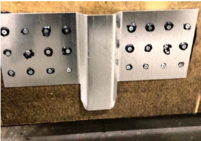
Image 15: Mounting brackets used on prefab panels by RC-panels (Source: R. Nuñez Larios)
