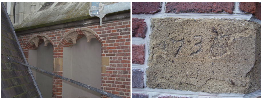
Figure 9. Blocks of Laacher tuff on the crossing tower of St. John's cathedral, 's-Hertogenbosch, dating back to the 1730's.
