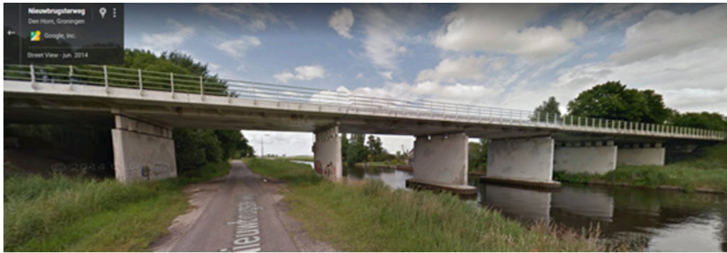
Fig. 5. Google Maps view of Nieuwklap Bridge.
