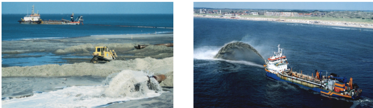
Figure 4.2. Trailing suction hopper dredgers pumping sand ashore (left; Roelse, 2002) and rainbowing sand (right; Hollemans, 2005).
