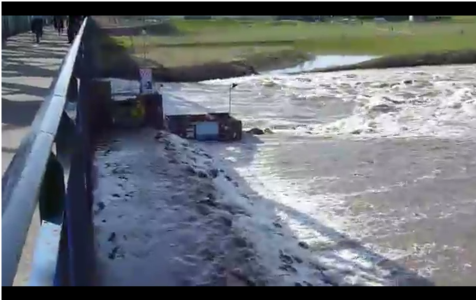
Figure 1.5: Extreme flow conditions with hydraulic jump through remaining opening of the weir, retrieved from: https://youtu.be/LvuxY0rYSXE
