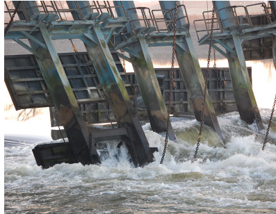
(a) Damaged weir
