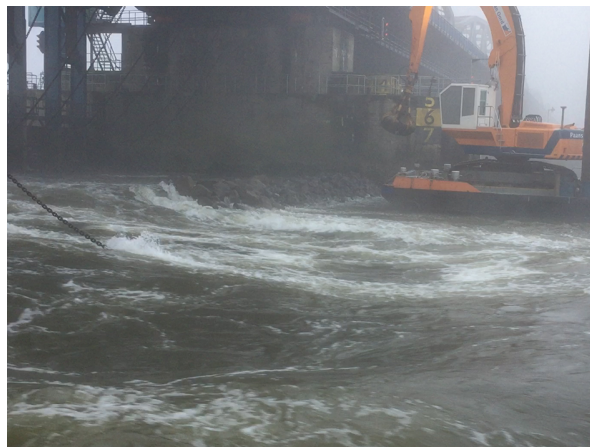
(a) Increased flow velocities during construction
