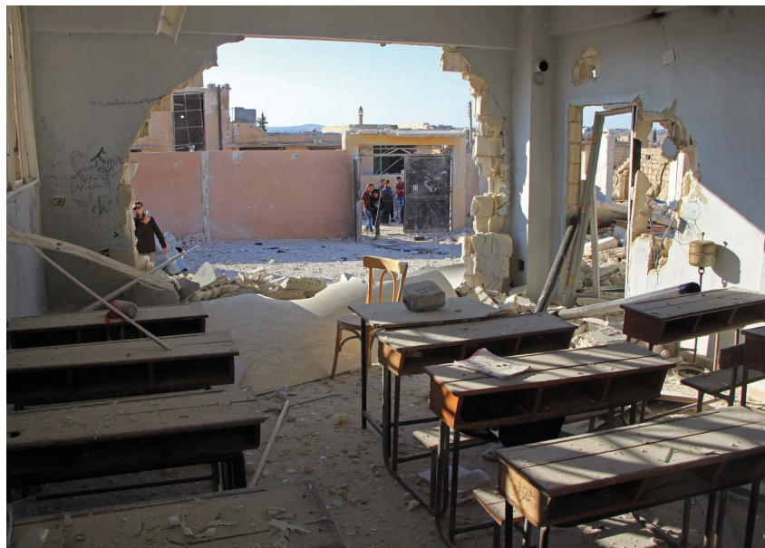
FIGURE 2. Destroyed school building in Syria. By: Omar Haj Kadour
