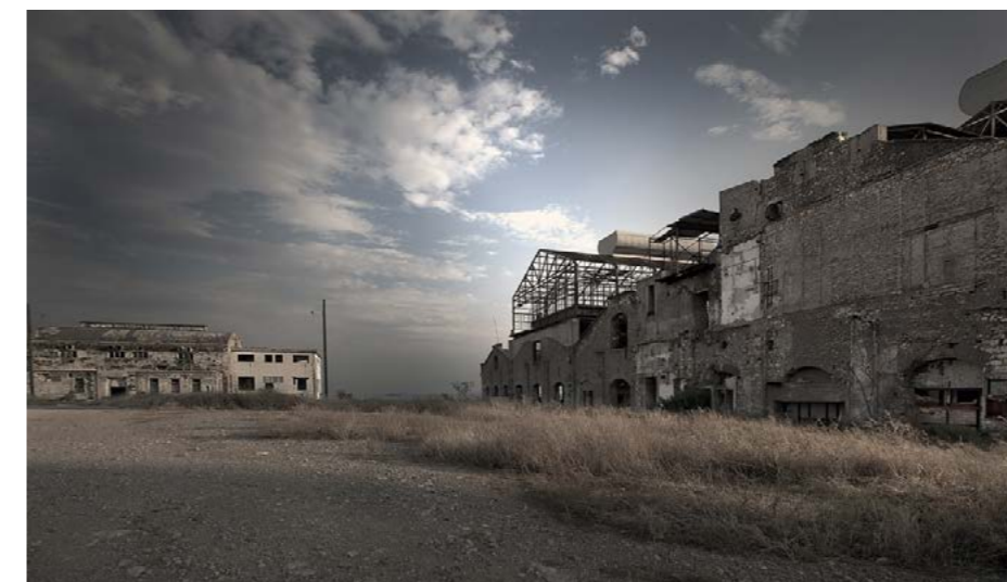
135. View of the remaining facilities of the fertilizers factory in Drapetsona .
