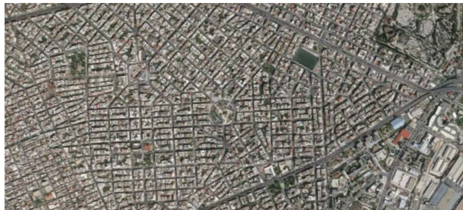
61b. Elements of cultural heritage as a result of the way the city has been formed.
