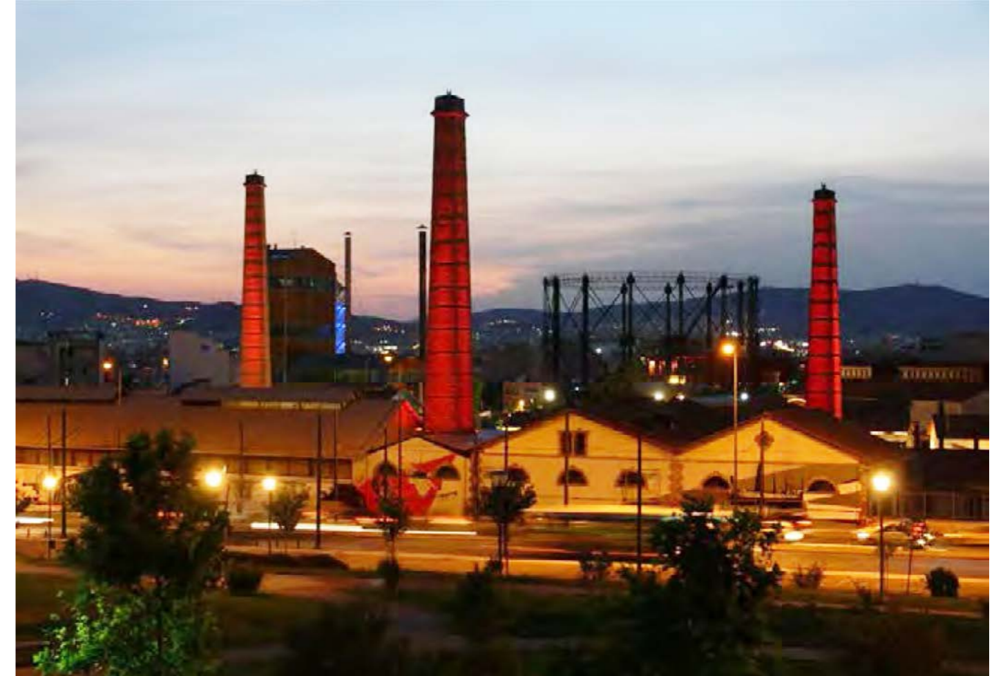
147. Technopolis Gazi- centre for culture and technology. The old factory after the renovation has become a famous destination for nightlife. The area around hosts from alternative theatres and underground bars to pop music scenes and fancy clubs. Source: Adrakta et al. (2005)
