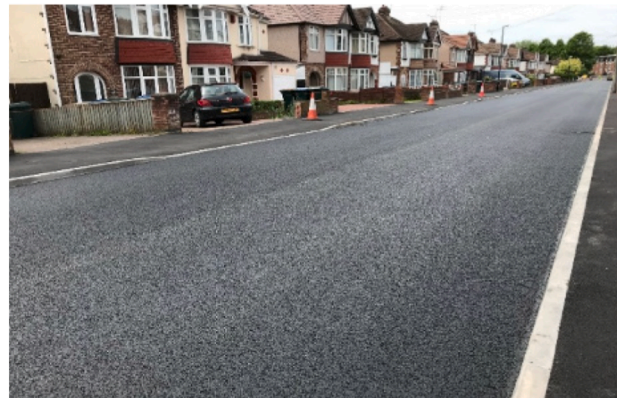
Fig. 6. Trial section with asphalt mixture containing waste plastic in Coventry City Council, UK [143].
