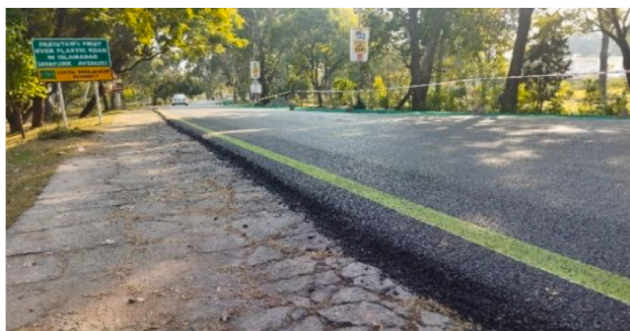
Fig. 7. Trial section containing waste plastic in Islamabad, Pakistan [158].
