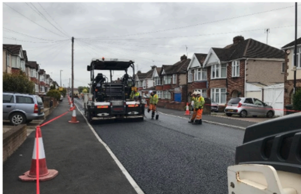
Fig. 6. Trial section with asphalt mixture containing waste plastic in Coventry City Council, UK [143].
