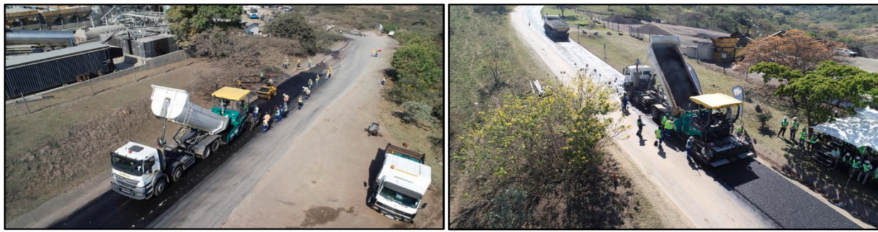
Fig. 8. Paving project having asphalt mixture containing recycled waste plastic in KZN province of South Africa [164].
