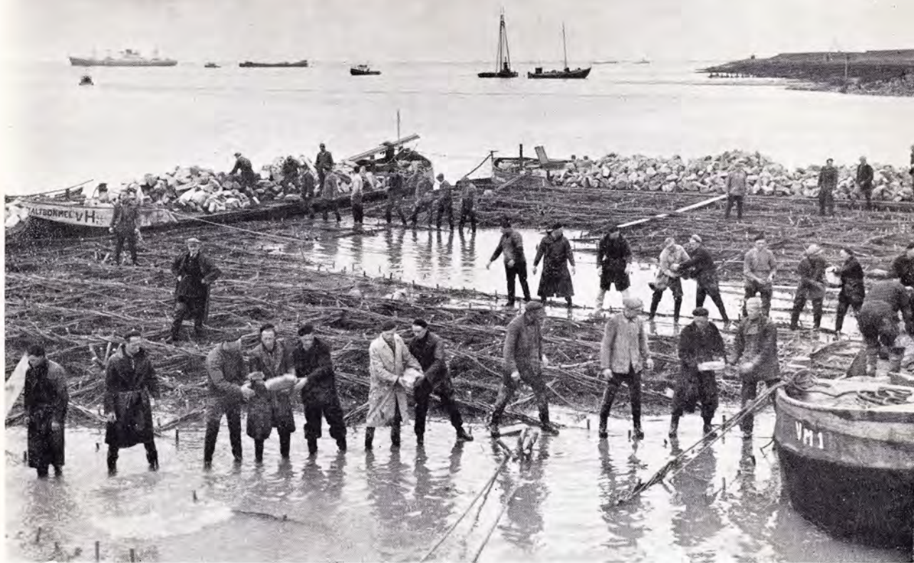
Defending the underwater parts of the shores of tidal waters by means of willow mattresses is a continuous business. Without these the lower parts of the Netherlands would be scoured away.
