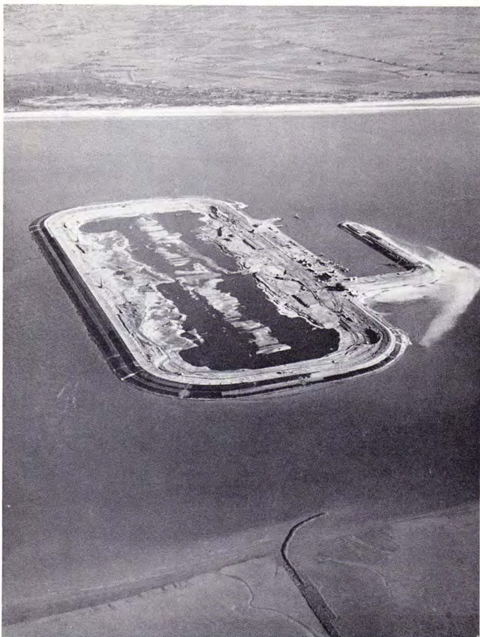
(Photo Stuwel.) The Delta works started in 1955 by closing off the main mouth of the Rhine, called Haringvliet. A sluice will be built in the central part of the tidal mouth, where a dike has been made encircling a building pit of about 250 acres. The sluice will be wide about 3500 ft. Dams to shut the remaining openings of the Haringvliet will be made after the sluice has been constructed.
