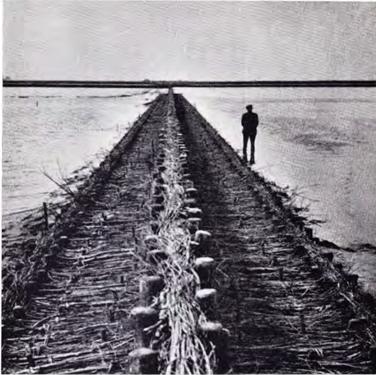
Long wooden groynes catch silt in the delta areas, so that land of sufficient height and great fertility is being gained.
