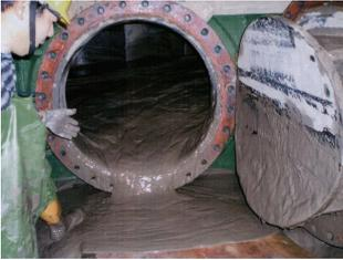
Figure 3.2: Mud accumulated in the penstock after typhoon Aere (2004). Courtesy of Hsu (2013)
