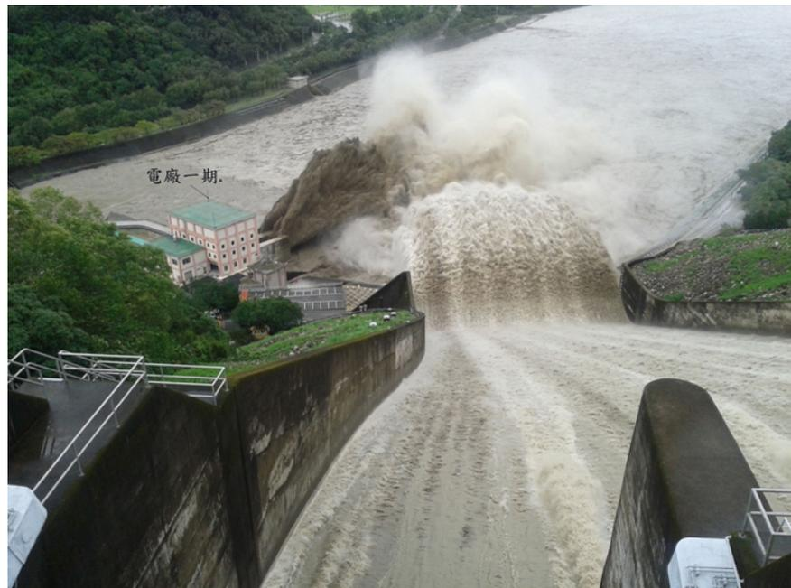
Figure 3.4: Mud concentrated flow from the silt-slucice and PRO turbine outlets, photo taken from the top of the spillway. Courtesy of <http://www.wra.gov.tw/>.
