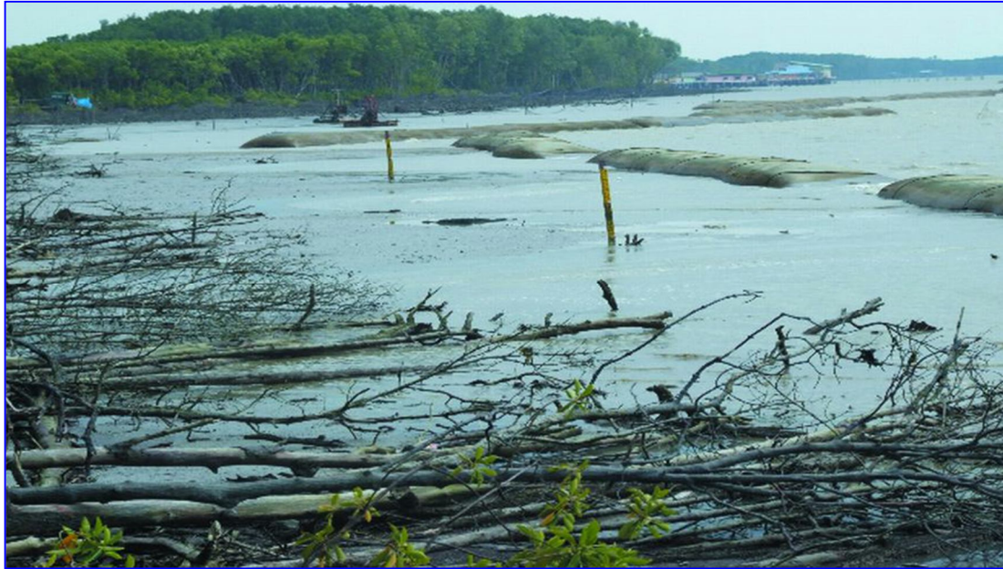
Figure 15 Geotextile tube breakwaters at Tanjung Piai with substrate build-up behind it (source: Tan, K.S. et al)
