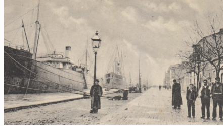
Fig. 11: View of Sulina port city 1900 Source: Wikimedia Commons, 2012
