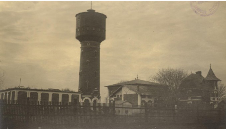
Fig. 14: Water Treatment Facility, 1951 Source: Adhristal, ResearchGate publication, n.d.
