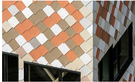
Figure 20: Steni up-cycled facade panels, Tullinløkka, Oslo (Source: https://omnisusa.com/projects/kristian-augusts-gate-13/# )
