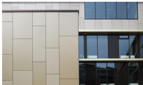
Figure 19: Phenolic panel façade design application (Source: www.trespa.com )
