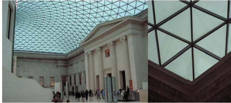
Figure 4.18: The Great Courtyard at the British Museum, London, UK; the right hand image shows a detail of the steel structure.
