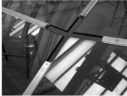
Figure 2.5: The connections in the faceted glass dome, from (Veer et al. 2003).
