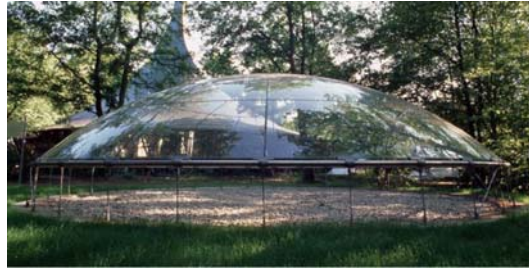
Figure 2.8: The frameless glass dome at the ILEK in Stuttgart, from (Blandini & Sobek 2005).
