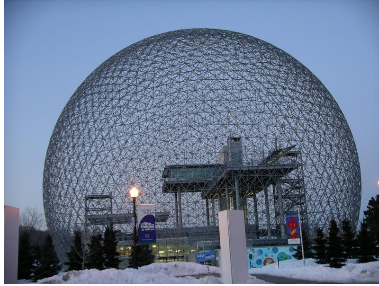
Figure C.1: The geodesic dome biosphere, built for the 1967 EXPO in Montreal, Canada. The dome represents 75% of a full sphere. ( 2007h)
