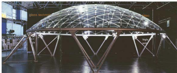
Figure 2.6: The glass dome by Seele GmbH at the Glasstec 1998, from (Behling & Behling 1999).
