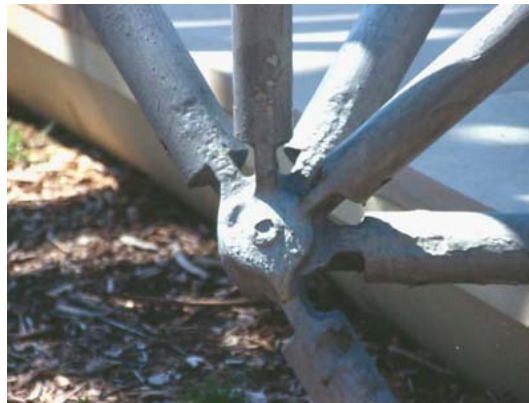
Figure 2.13: A node in the dome structure ( 2007c)
