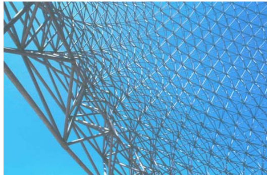
Figure 2.12: A view on the space frame forming the structure ( 2007c)
