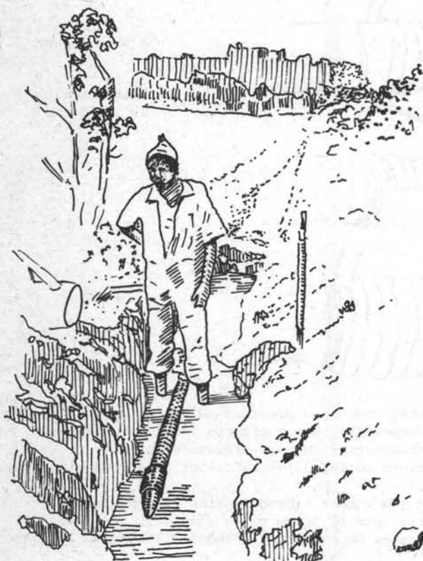
figure 21. Repair of bamboo pipeline.
