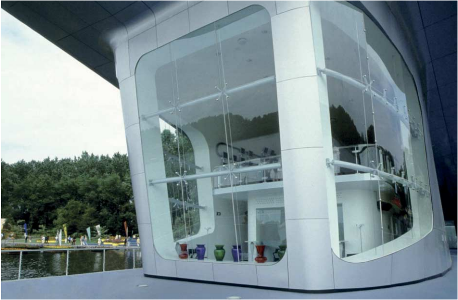
FIG. 126 Cold deformed glass panels in the South facade
