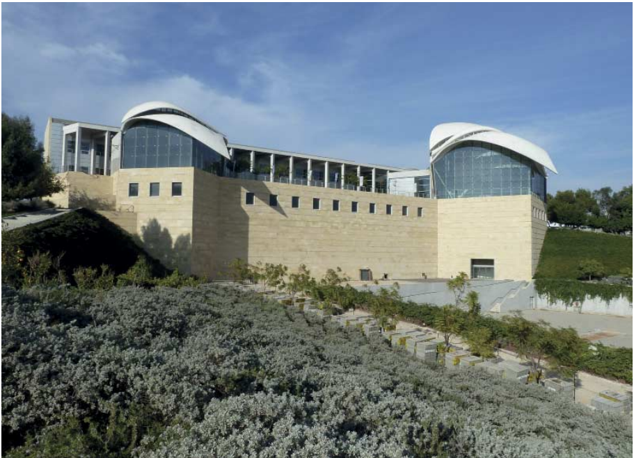
FIG. 86 Overview of the building site after completion.
