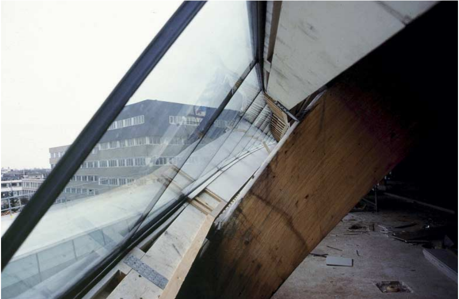
FIG. 55 Detail of the 'spaghetti' glass strips with cold twisted glass
