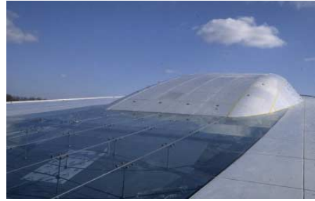
FIG. 32 Completion of the roof
