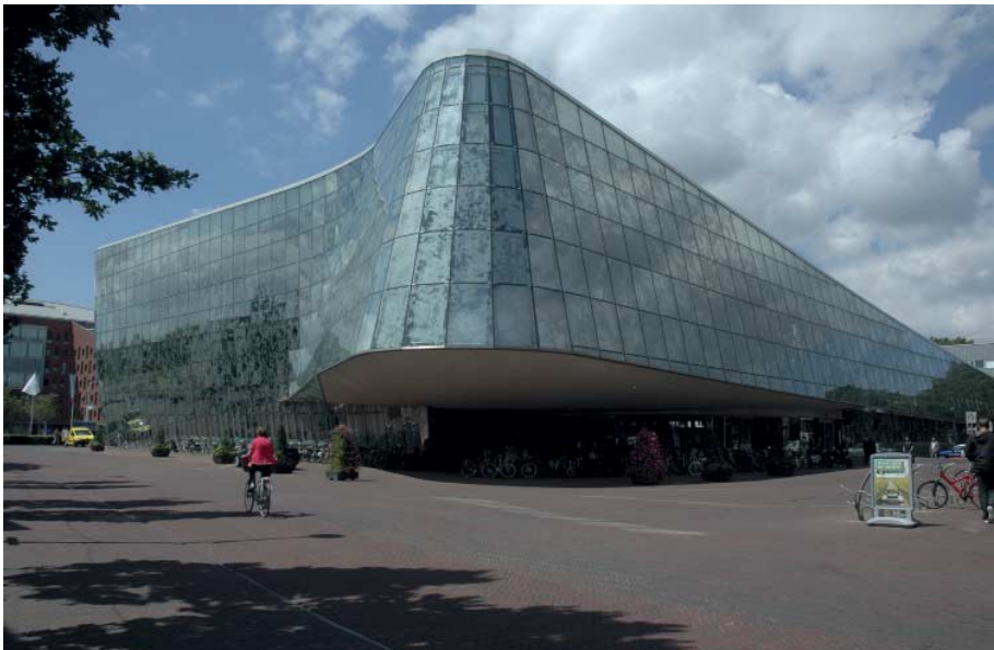
FIG. 46 The front façade after completion
