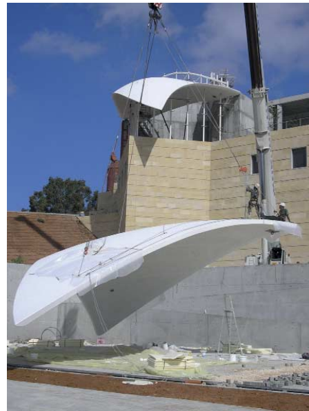
FIG. 84 Preparation and hoisting of the upper and lower wing of the Library in August 2005.
