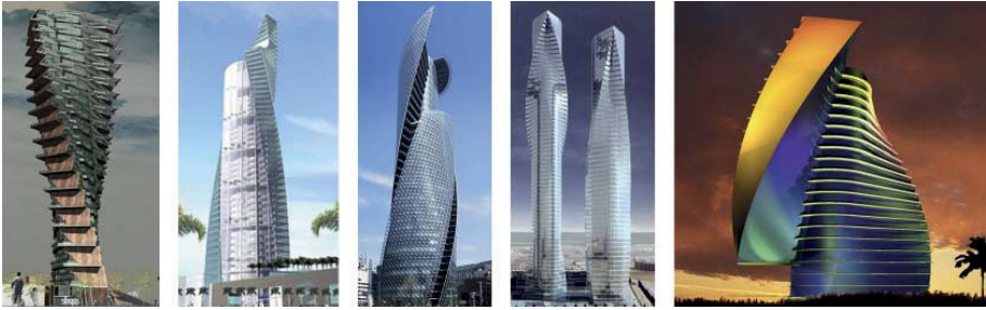
FIG. 99 Different basic twisted high rise towers: Urban Totem, Mississauga, Canada [by Donner&Sorcinelli]; Kuwait Trade Centre, 2009 (by NORR); Mode Gakuen Spiral tower, Nagoya, Japan, 2008 (by Nikken Sekkei); Torre Alicante and Torre Valencia, Valencia, Spain [by Calatrava]; Sea Breeze tower, Dubai [by author]
