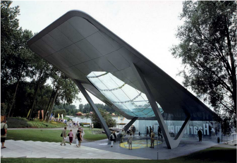
FIG. 127 Glass pond at the entrance of the Municipal Floriade Pavilion
