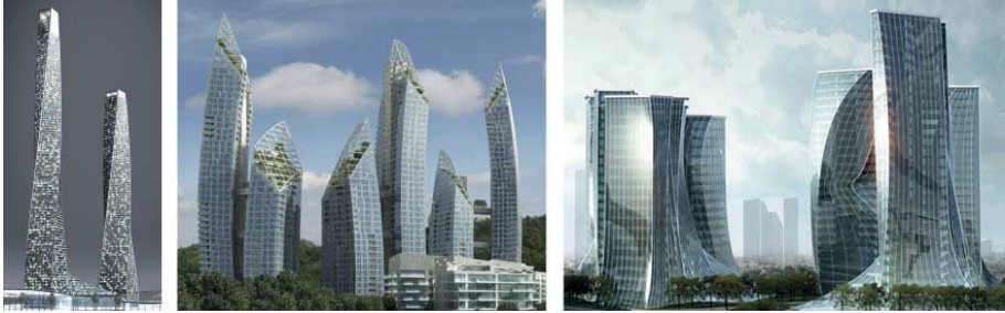
FIG. 107 Dubai Towers, Istanbul, proposed [by Inhouse Design]; Caribbean, Keppel Bay, Singapore [by Libeskind]; Dostyk Business Centre, Almaty, Kazakhstan [by NBBJ].
