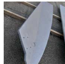
FIG. 140 Twisting web member spanning between primary frames: a steel sheet folded across its diagonal
