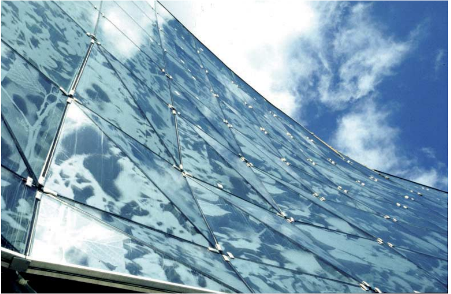
FIG. 130 Detail of the warped Front façade of the Town Hall
