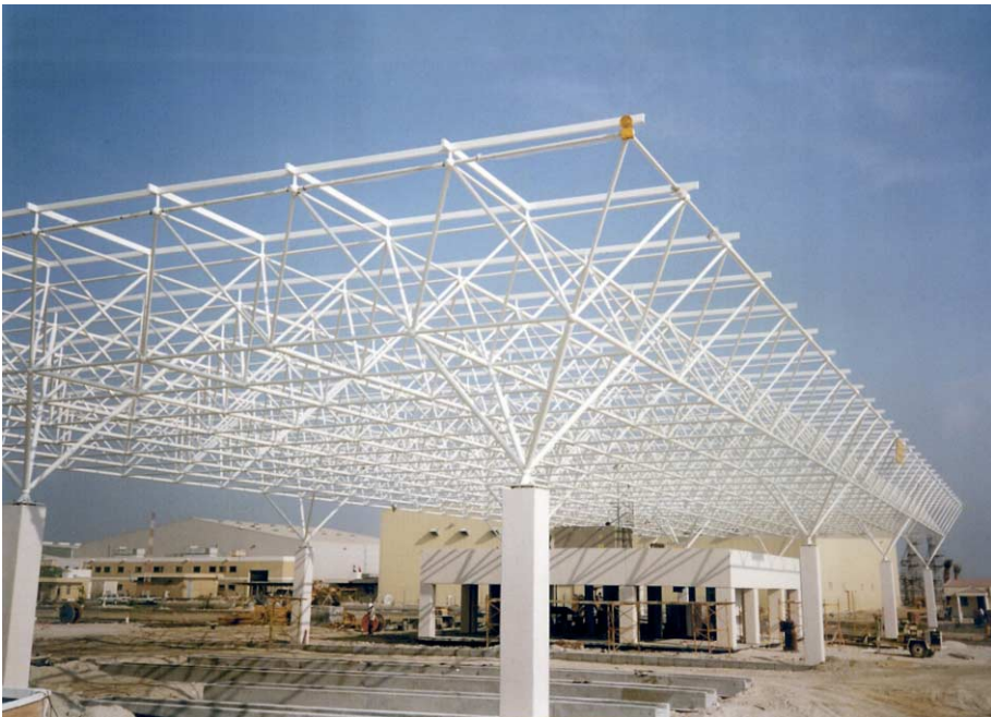
FIG. 02 Space structures (Air India hangar in Dubai during construction)
