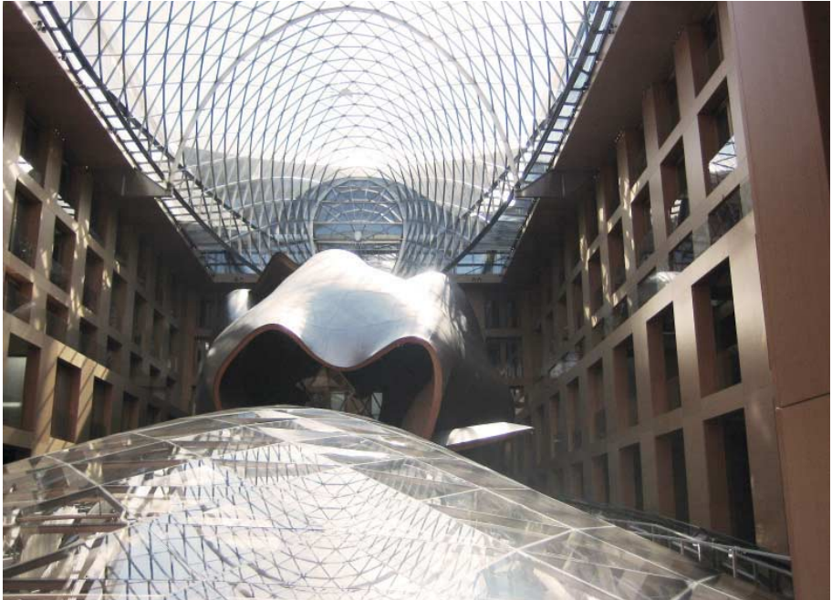
FIG. 24 Interior of the DG Bank
