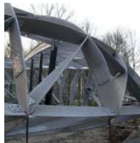
FIG. 139 The primary structure consists of planar frames
