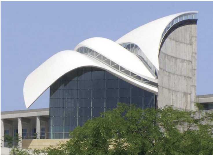
FIG. 133 The Great Hall just after installment of the composite sandwich roofs in November 2005
