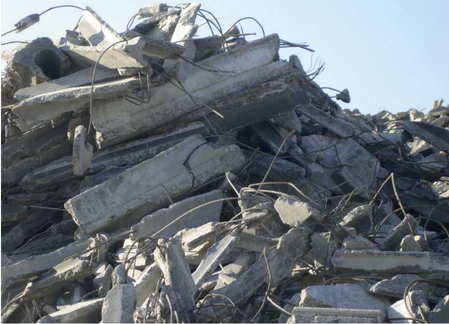
FIG. 17 Pulverizing a decent building should be avoided: capital investments go from 100% to 3%. The gravel is used for making-concrete again
