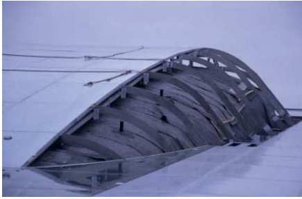
FIG. 31 Opening for the bent panels
