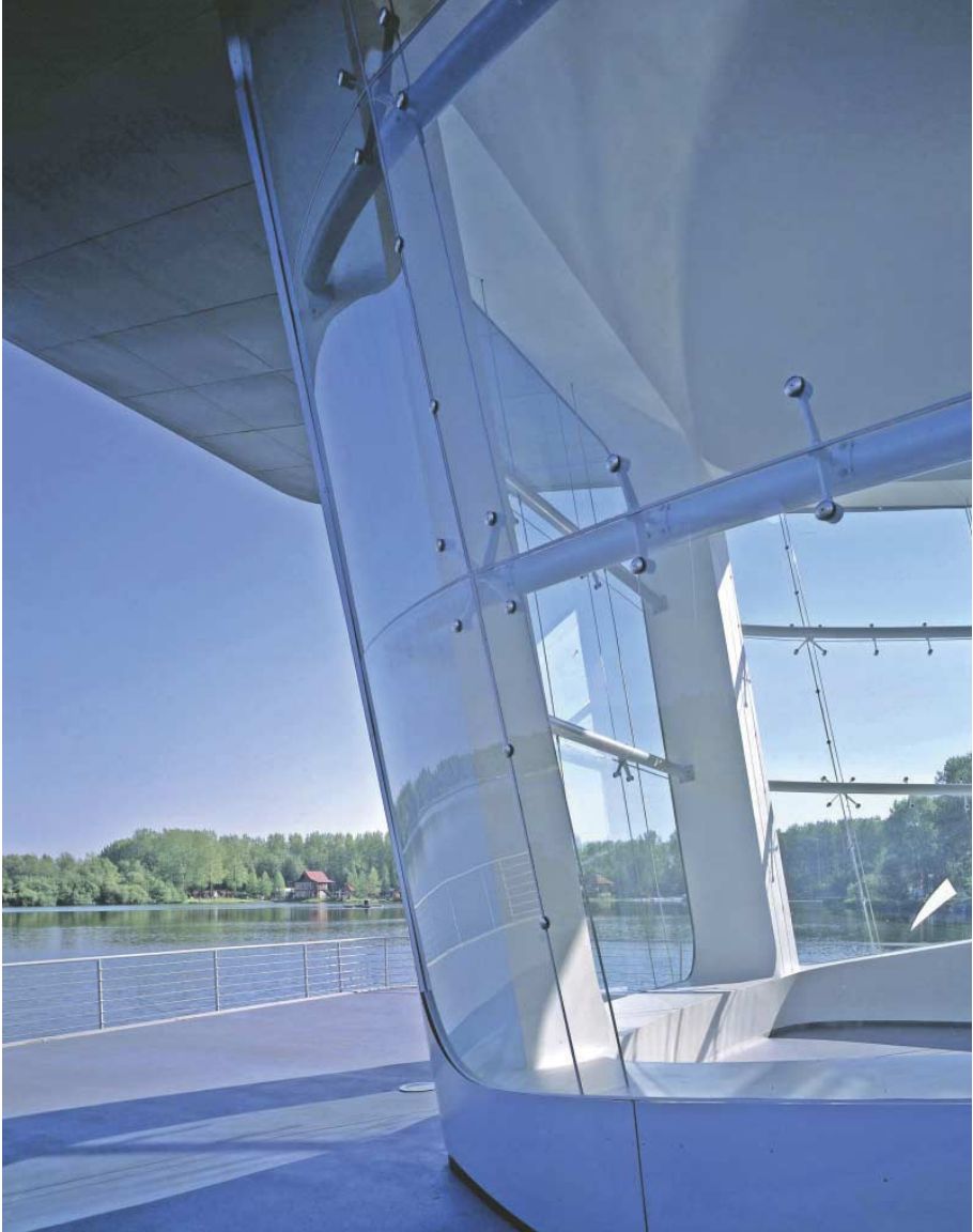
FIG. 38 Cold bent glass with fixing nodes.
