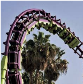
FIG. 141 Tubular rollercoaster-track with 3D-curved backbone. [Image courtesy www.coastergallery.com ]
