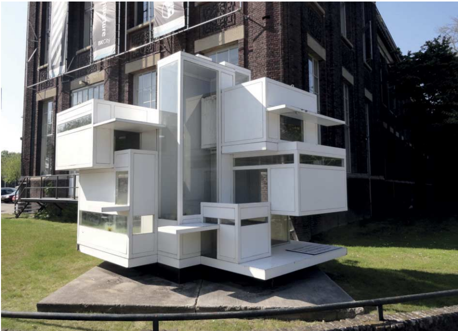
FIG. 06 Prototype of Maison d'Artise 1923, realized at TU Delft 2003 by students, but originally one of the first designs of a new architectural style, boosted by the technical developments of reinforced concrete floor slabs and watertight bituminous roofing in the 1920s
