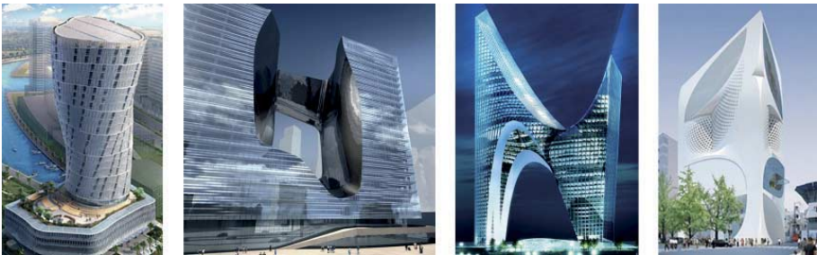
FIG. 100 Different examples of 'merger' type high rise buildings: Iris Crystal, Dubai, planned [by Aedes]; Opus, Dubai, -2010 [by Hadid]; Gazprom, Petersburg [by Herzog & de Meuron]
