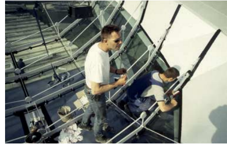
FIG. 34 Assembly of the dot-shaped suspensions
