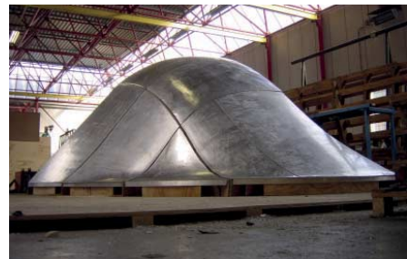
FIG. 30 Completion of all bend panels for one side
