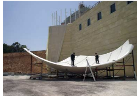
FIG. 83 Assembly of the roof segments by gluing and bolting glass fibre polyester plates on the seams before applying the finishing layer.
