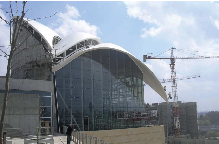
FIG. 88 Finishing of the top layer of the roof by "airborne builders"
