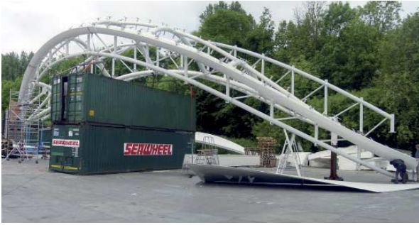
FIG. 77 The central body of the Great Hall (spanning ca. 30m).
