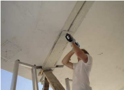
FIG. 83 Assembly of the roof segments by gluing and bolting glass fibre polyester plates on the seams before applying the finishing layer.
