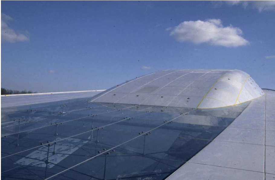
FIG. 128 Roof panels created with Exploform technique after installation
