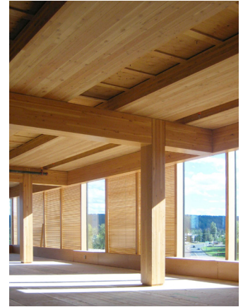
Load-bearing timber structure
