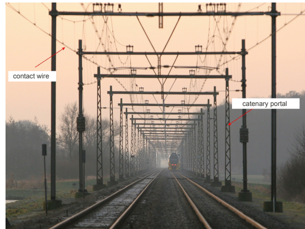
Figure 2.12: Catenary system
