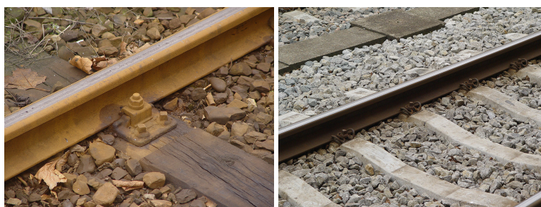
Figure 2: Timber sleeper (left) and concrete sleepers (right)
