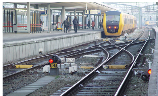
Figure 1: Cross-over (K) between two sets of switches (W)
