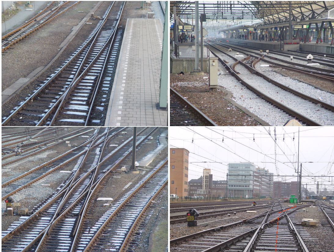
Figure 2.15: Different switch types, from top and from left to right: normal switch, coupled switches, entire Englishman, half Englishman (the red arrows indicate the impossible direction)
