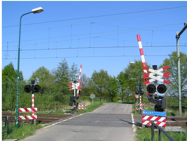
Figure 2.9: Protected level crossing
