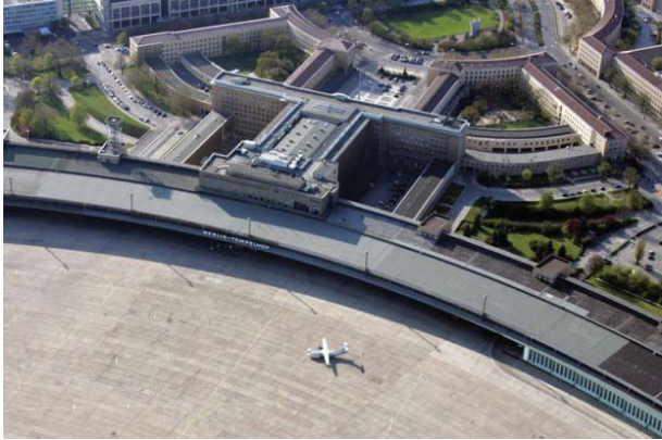
Figure 27 | Tempelhofer Feld terminal (by DDP)
