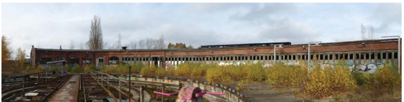
Figure 59 | Picture of the main building of the railway yard (by author)
