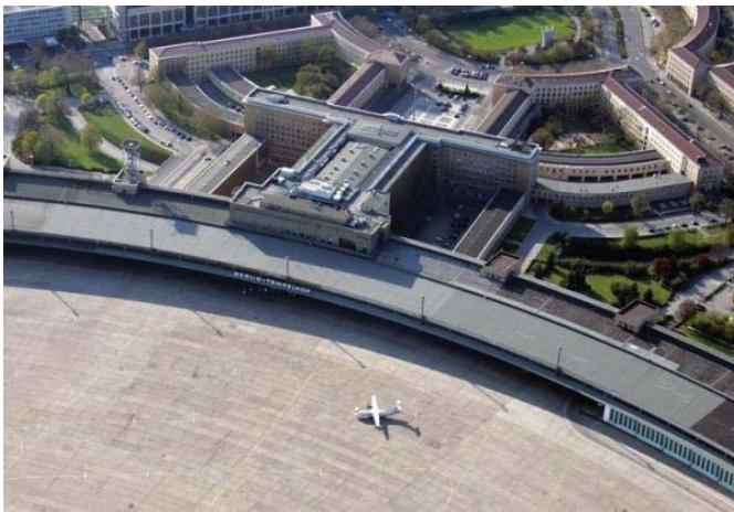
Figure 44 | Tempelhofer Feld terminal (by DDP)
