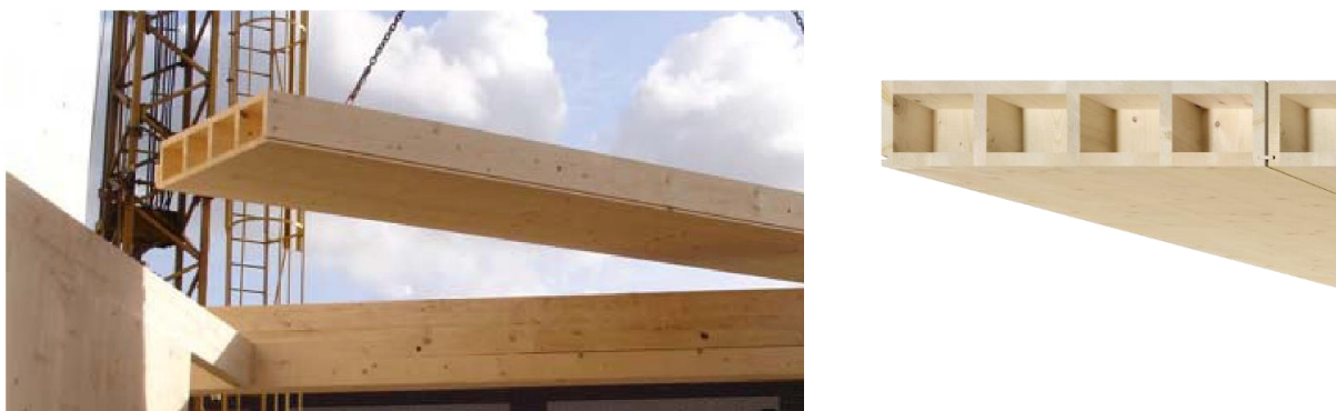
Figure 25: Lignatur, left (den Boon & Fraanje, 2007), right (Lignatur, 2019)
