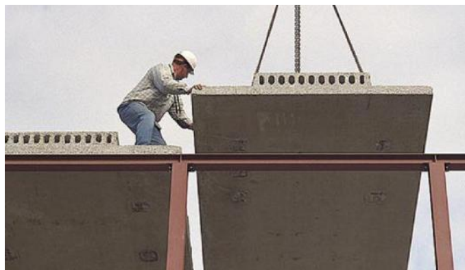
Figure 16: Wing floor (den Boon & Fraanje, 2007)
