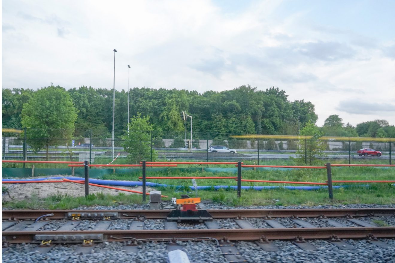
Railway cutting through the forest
