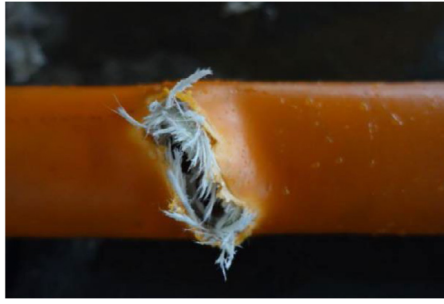
Fig. 15. Detail of a burst position.
