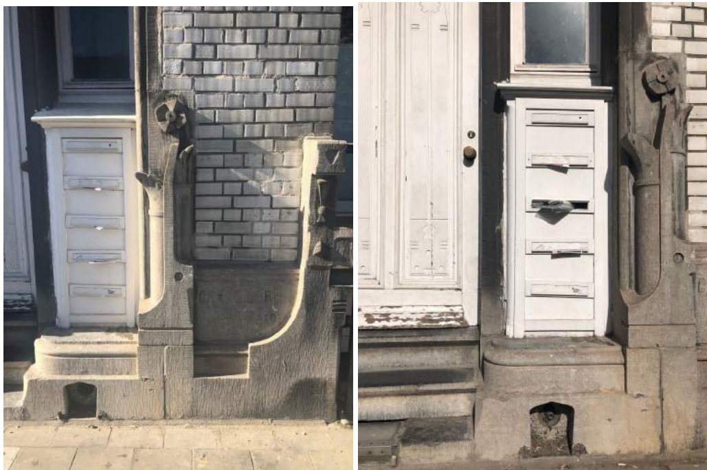
Fig. 19 | Comparison of the same elevation made of limestone elements when it is in sun and in shadow. Because of sculptural qualities of limestone it is very easy to shape it into blocks, bricks, and even into ornamentation.
