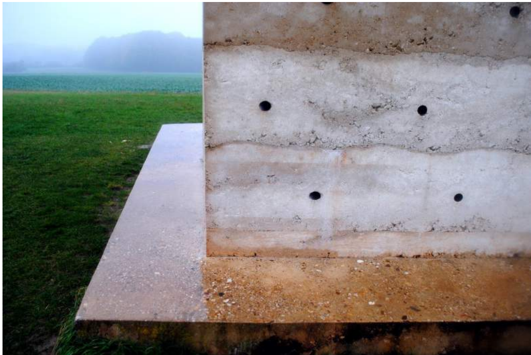
Fig. 14 | Tamped concrete in Bruder Klaus field Chapel near Wachendorf (Peter Zumthor). Photographs: Dr. Leeke Reinders
