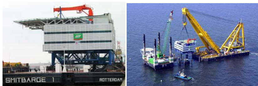
Figure 2.3: Left: Offshore substation. Right: Installation of offshore substation.
