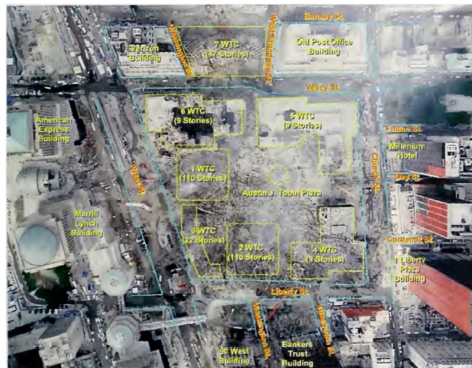
Fig.27 Aerial view after the collapse of all WTC buildings. (NIST, 2005).
