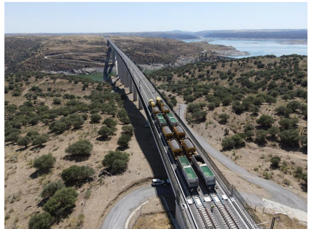
Figure 6. Load testing at El tajo Viaduct.
