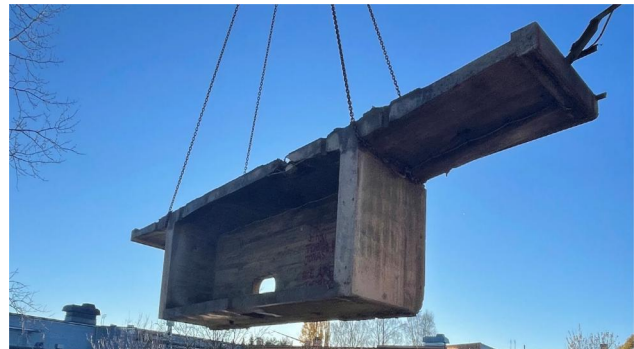
Figure 17. A section from the kalix bridge conserved for further testing.
