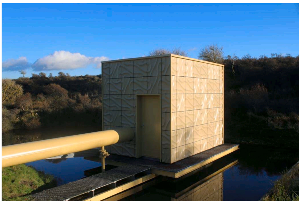
Fig. 3. Façade panels applied at the pumping station in a natural reserve [picture from D1.9 WIDER UPTAKE report].
